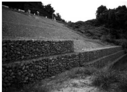
< 盛土のり尻補強 >
