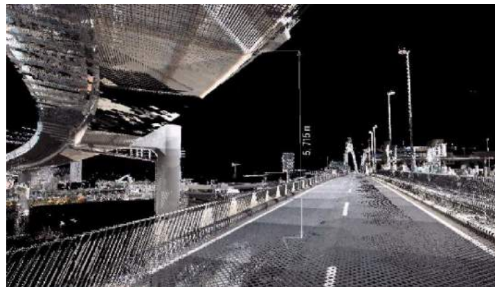
Figure 4. Clearance check on point cloud.
