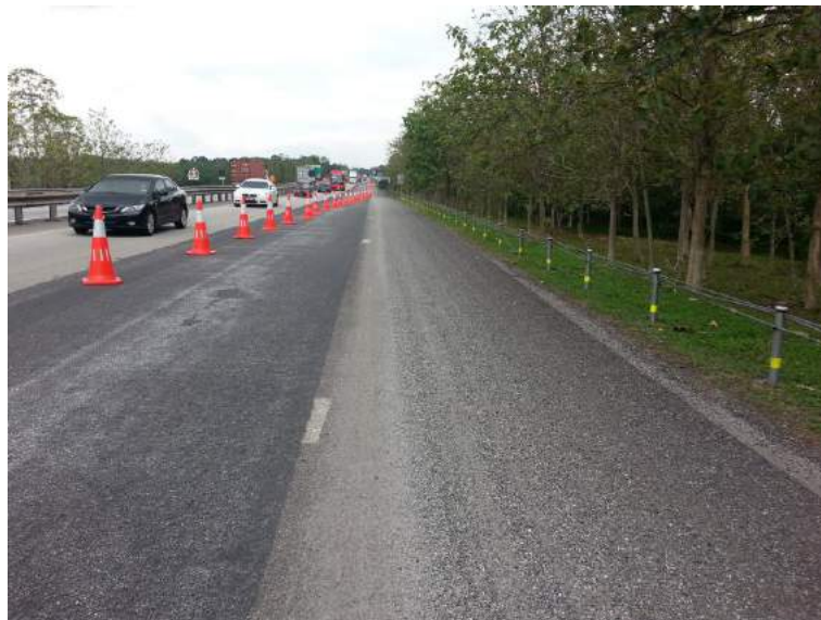
Figure 6. Ravel off micro surfacing surface
