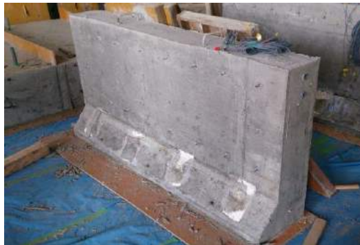
(c) Completed Hollow RC Barrier
