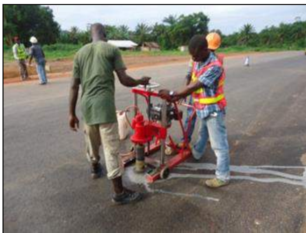
Figure 8: Post Construction Testing
