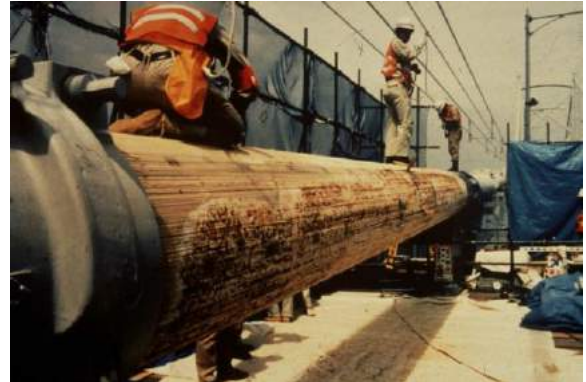
Figure 4. Unwrapped Cable at Innoshima Bridge
