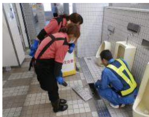
Figure 18: Checking a drain for odor
