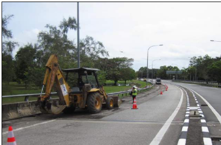
Figure 3. Milling process to scrape-off the existing asphalt layers
