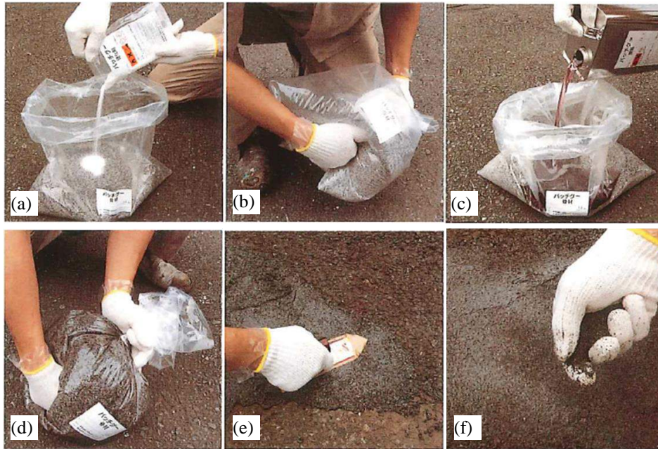
Figure 16. Application method for resin-type road surface repair material: (a) Adding the curing agent to the aggregate, (b) Mixing, (c) Adding the resin, (d) Mixing, (e) Spreading and leveling, and (f) Spreading anti-slip sand
