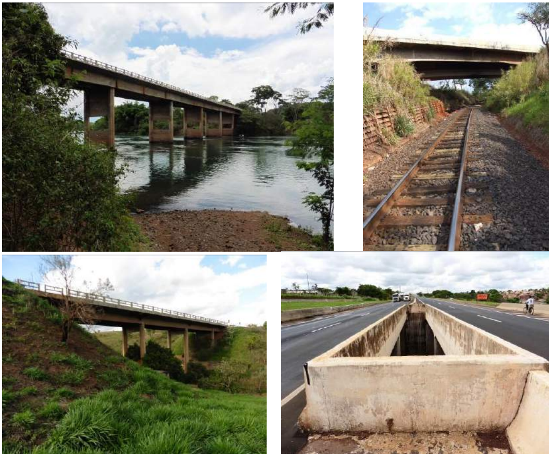
Figure 4. Some examples of the bridges to be upgraded
