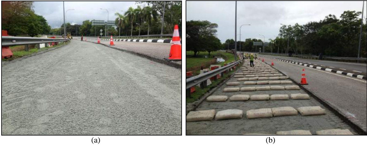
Figure 4. (a) Spread layer of quarry dust; and (b) positioning of cement and alkaline compound packaging to ensure an evenly distribution over the stabilized area
