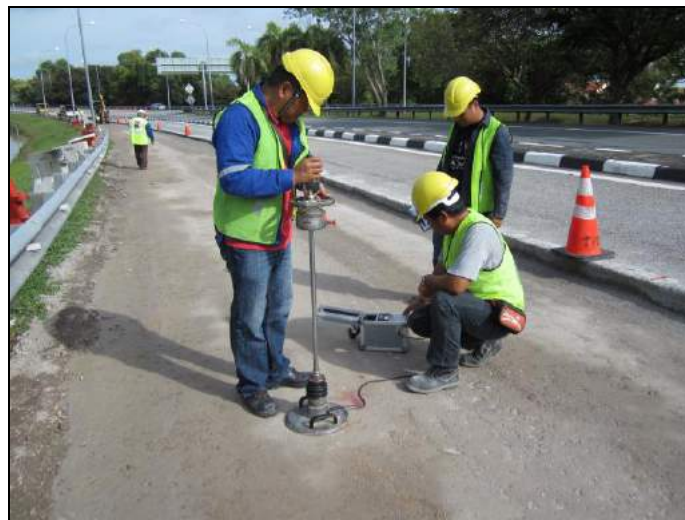
Figure 7. In-situ practical of Light Falling Weight Deflectometer (LFWD) test
