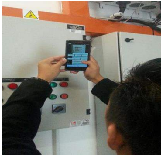
Figure 5: Asset Registration of M&E Components
