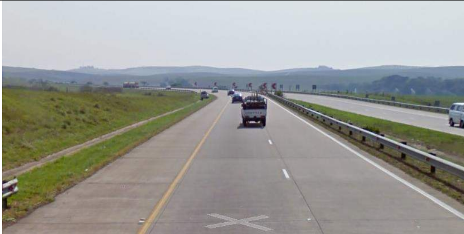
Figure 7. Mvoti River Bridge (North facing)
