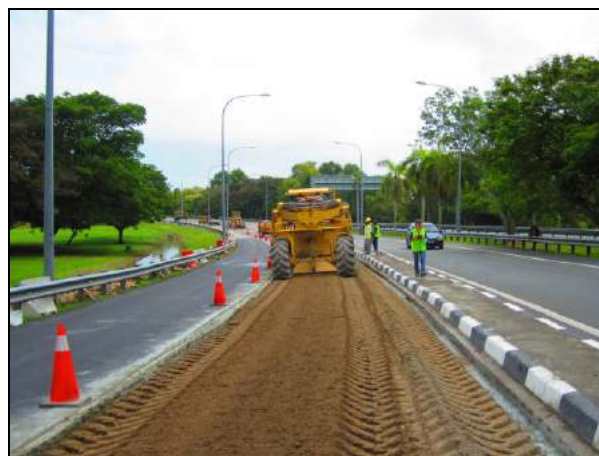
Figure 5. Mixing process of mixed soil-OPC-alkaline compound by special rotary mixer machine, CAT RM500
