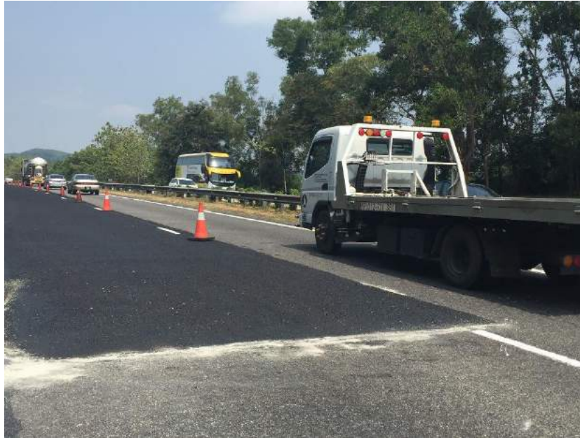
Figure 3a. Good quality transverse joint
