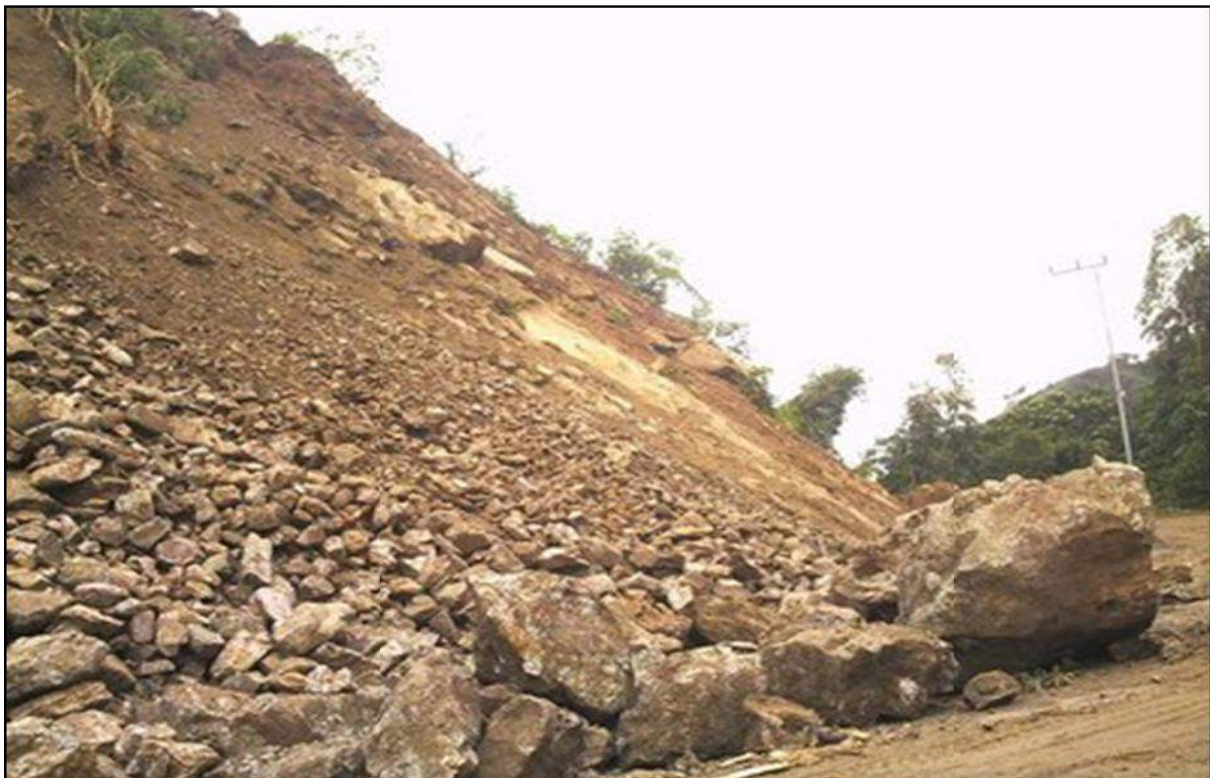
Figure 2. Avalanched Debris Falls at KM 13+000 Ende, trans road Ende – Maumere, East Nusa Tenggara Provinces (IRE, 2008)
