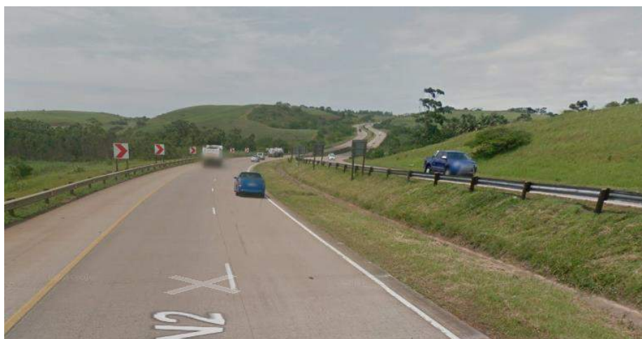
Figure 6. Umhlali River Bridge (South Facing)
