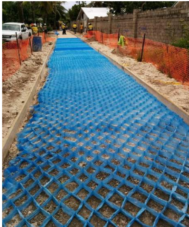
Figure 5. Geocell formwork expanded and tensioned and ready for placement of concrete.
