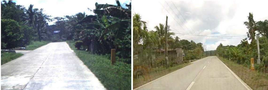
KM831 (left = before upgrade; right = after upgrade)
