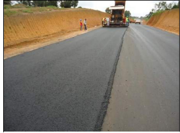
Figure 11: Common Worksite Traffic Management.
