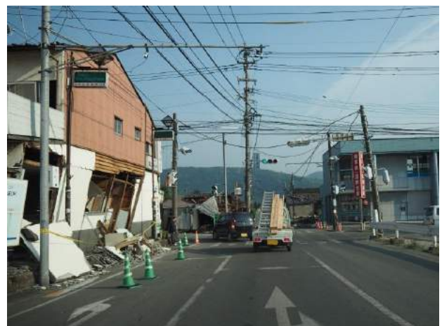
Figure 9. House collapse at Mashiki Town
