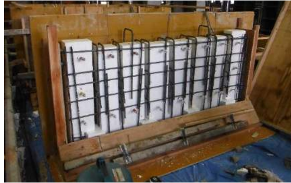
(b) Hollow RC Barrier inside of Styrene foam
