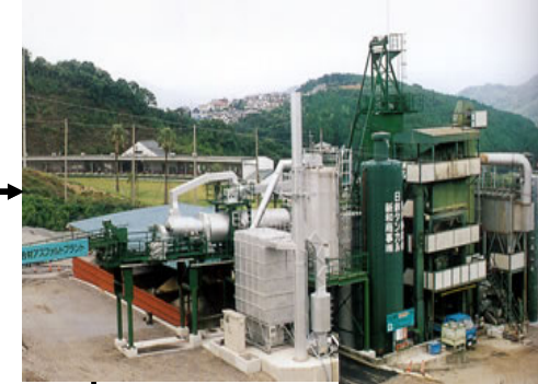
Asphalt Mixture Recycle Plant
